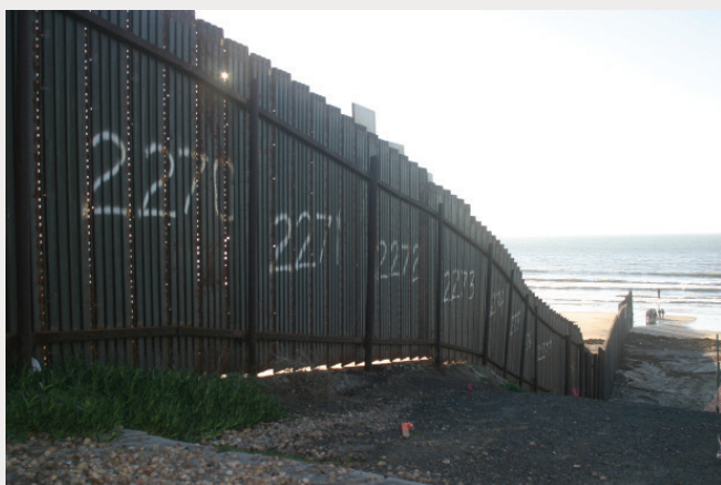
Landing mat border wall entering the Pacific Ocean south of San Diego. 2008. Scott Nicol.
