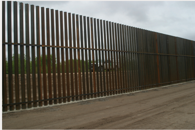
Border Patrol driving on flood control levee behind bollard border wall in El Calaboz, Texas. 2009. Scott Nicol.
