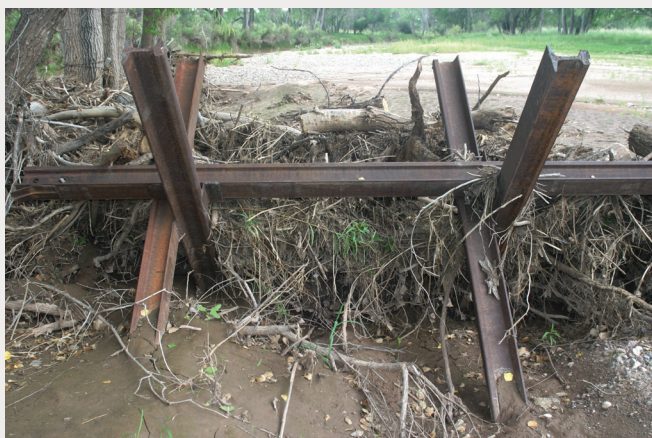
Vehicle barrier trapping debris in the San Pedro River. 2012. Scott Nicol.
