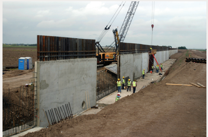
Levee-border walls under construction in south Texas. 2008. Scott Nicol.
