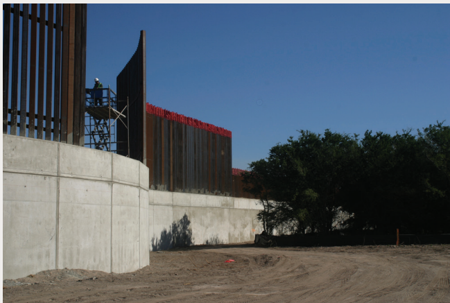
Levee-border wall under construction in Hidalgo, Texas. 2009. Scott Nicol.
