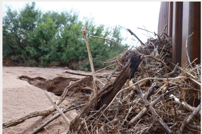
Debris and sediment backed up against a bollard border wall in the San Pedro Riparian National Conservation Area. 2012. Wendy Burke-Ryan.
