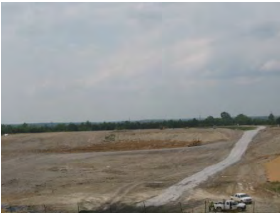
Active disposal cell at the Arrowhead Landfill in Uniontown, AL
